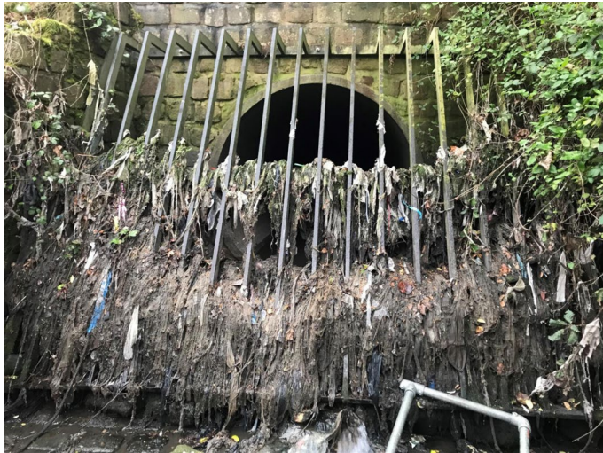
Fig. 2 | An outfall from a CSO on the River Tame in Greater Manchester, UK. Figure reproduced with permission from ref. 25, Springer Nature Limited.
