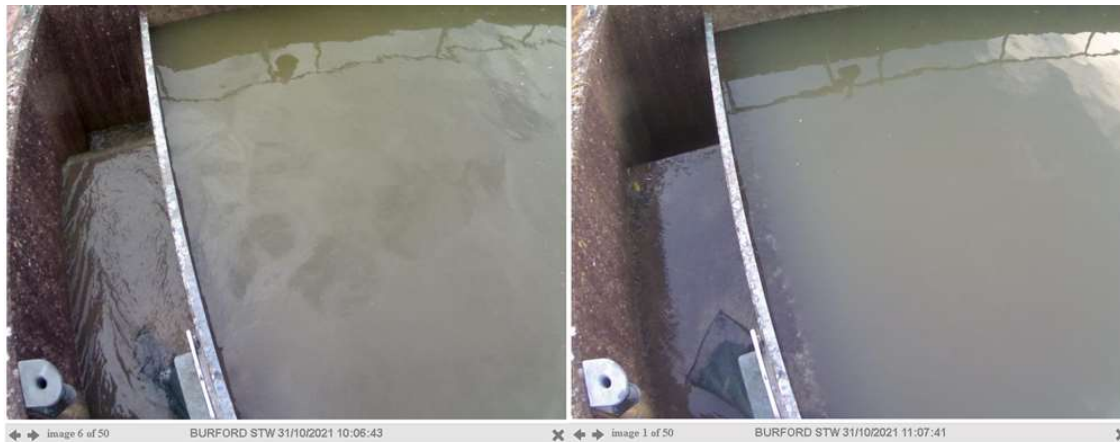
Figure 3: time lapse photographs of Burford STW's storm tank and EDM monitor (bottom left corner) recording an unreported and undetected spill
